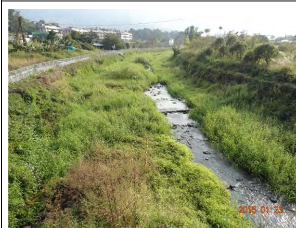
Photo 5: River channel and gabion colonized by vegetation (Middle Section).
