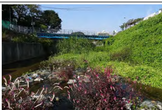
Photo 4: Gabions and River bed (Middle section)
