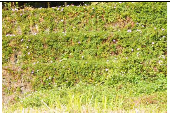
Photo 4: Gabions and River bed (Middle section)
