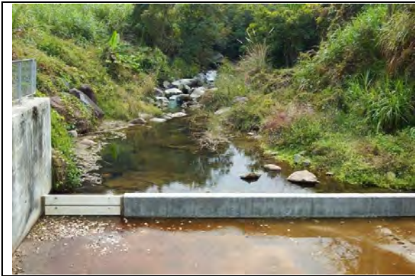
Photo 1: General view of the reference site
