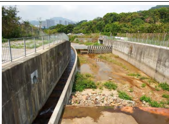
Photo 2: General view of the river channel (Upper section)
