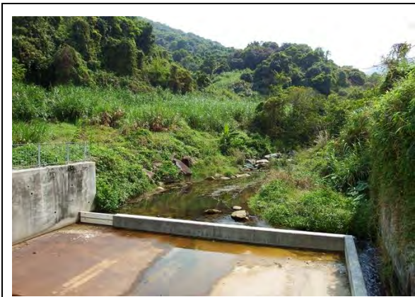
Photo 1: General view of the river channel (Reference site)
