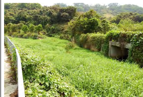
Photo 3: General view of the river habitat (Upper section).
