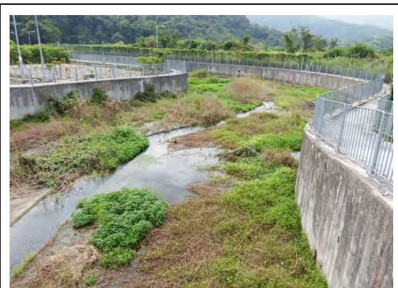
Photo 2: General view of the river habitat (Middle section).
