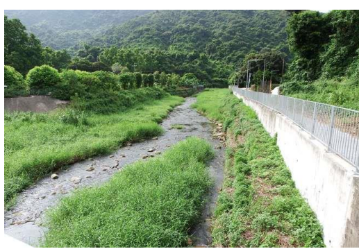
Photo 3: Dense vegetation coverage in Lam Tsuen River
