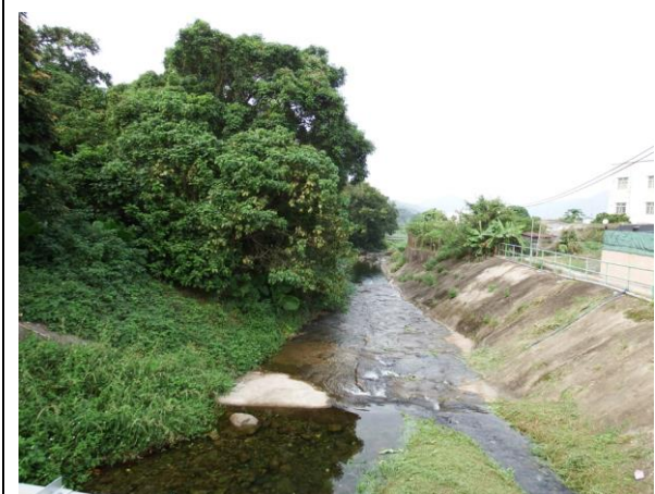
Photo 3: General view of the river (Upper section)
