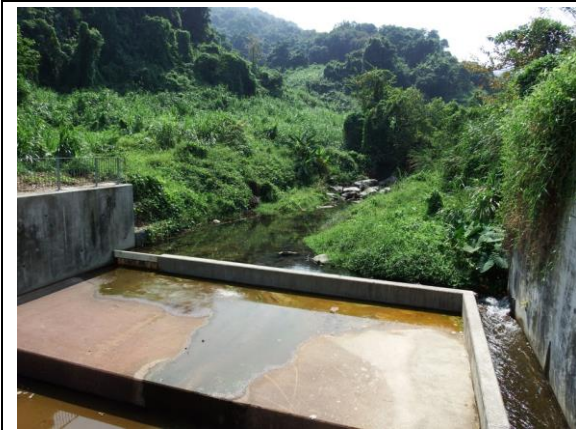
Photo 1: General view of the river channel (Reference site)
