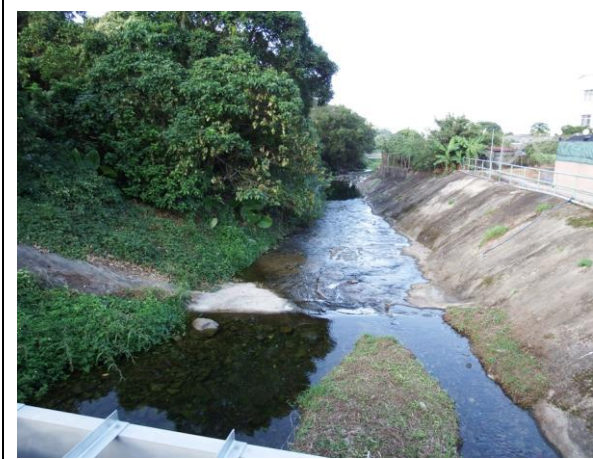
Photo 3: General view of the river (Upper section)
