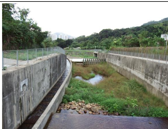
Photo 2: General view of the river channel (Upper section)
