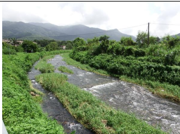
Photo 2: General view of the river (Middle section)
