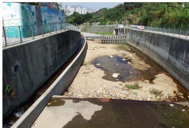
Photo 2: General view of the river channel (Upper section)
