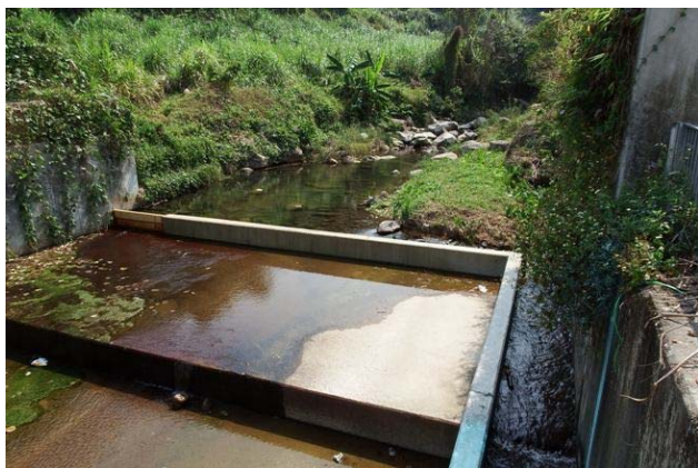
Photo 1: General view of the river channel (Reference site)
