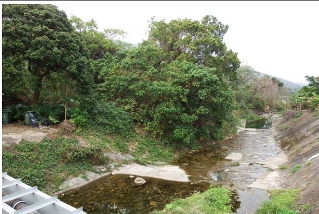
Photo 3: General view of the river (Upper section)
