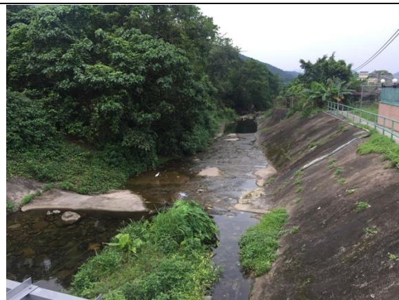
Photo 3: General view of the river (Upper section)
