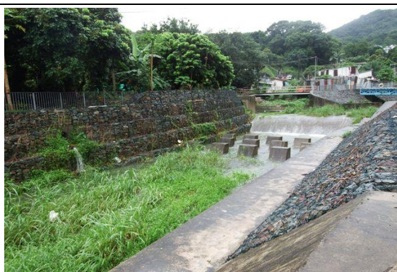
Photo 4: Vegetation sparsely growing on gabion (Middle section)
