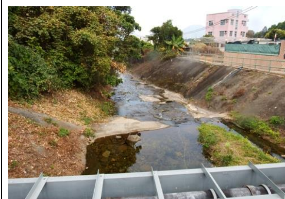
Photo 3 : General view of the river (Upper section)
