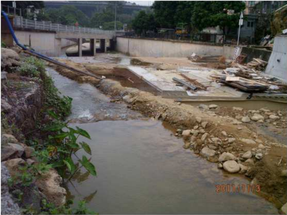
Fig.6.2 – The river quality was acceptable with no muddy water observed (photo provided by Contractor).
