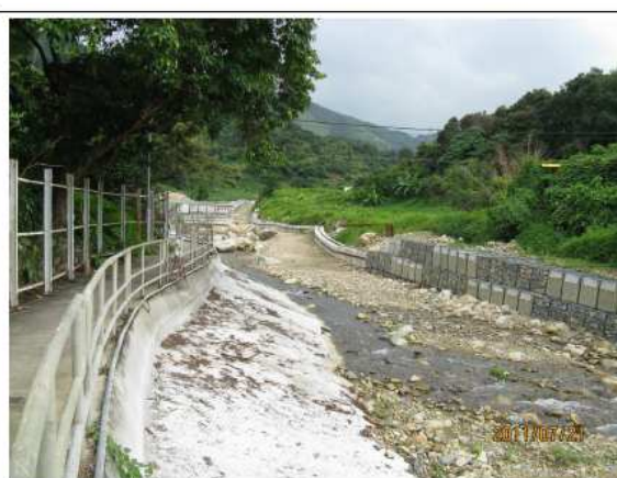
Photo 2: General view of the works area
