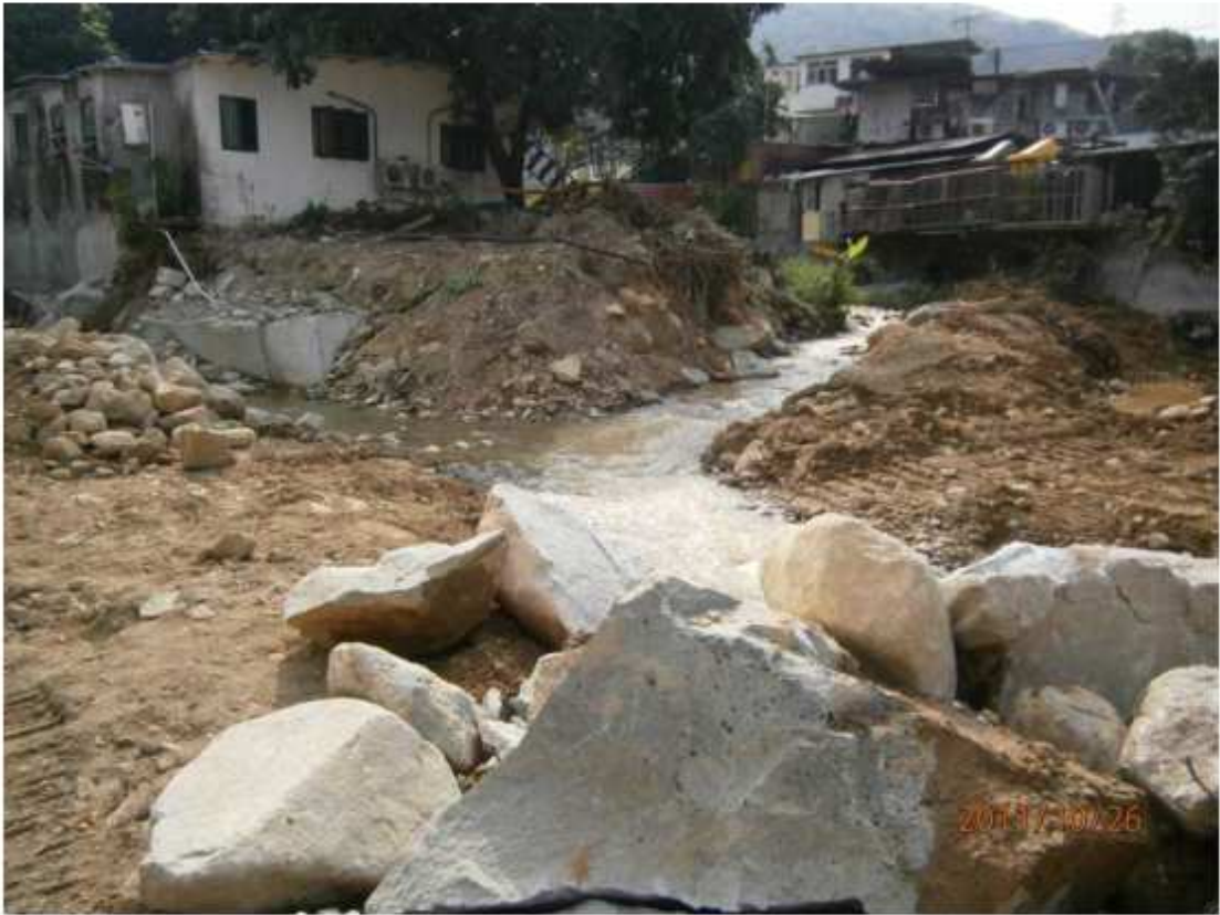
Fig.2.2 –Seepage of untreated site water directly into the river.
