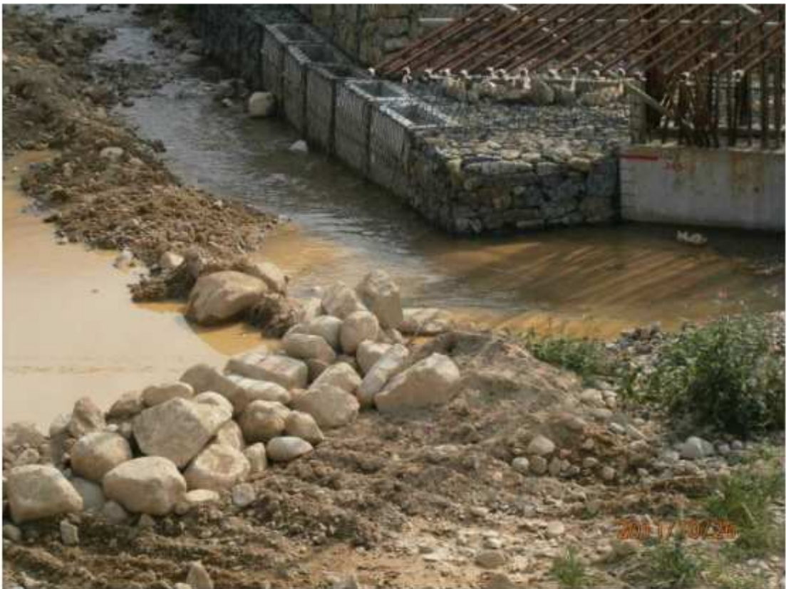
Fig.2.2 –Seepage of untreated site water directly into the river.
