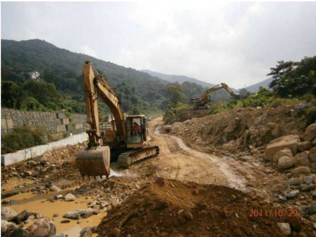
Fig.4.2 – Muddy water was generated from river diversion work.
