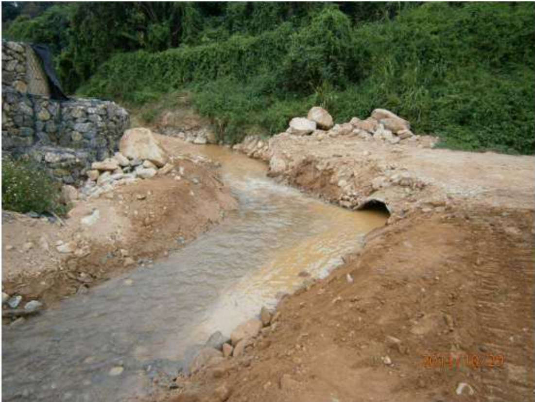
Fig.4.2 – Muddy water was generated from river diversion work.
