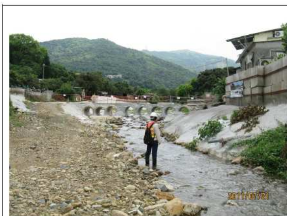
Photo 1: General view of the works area
