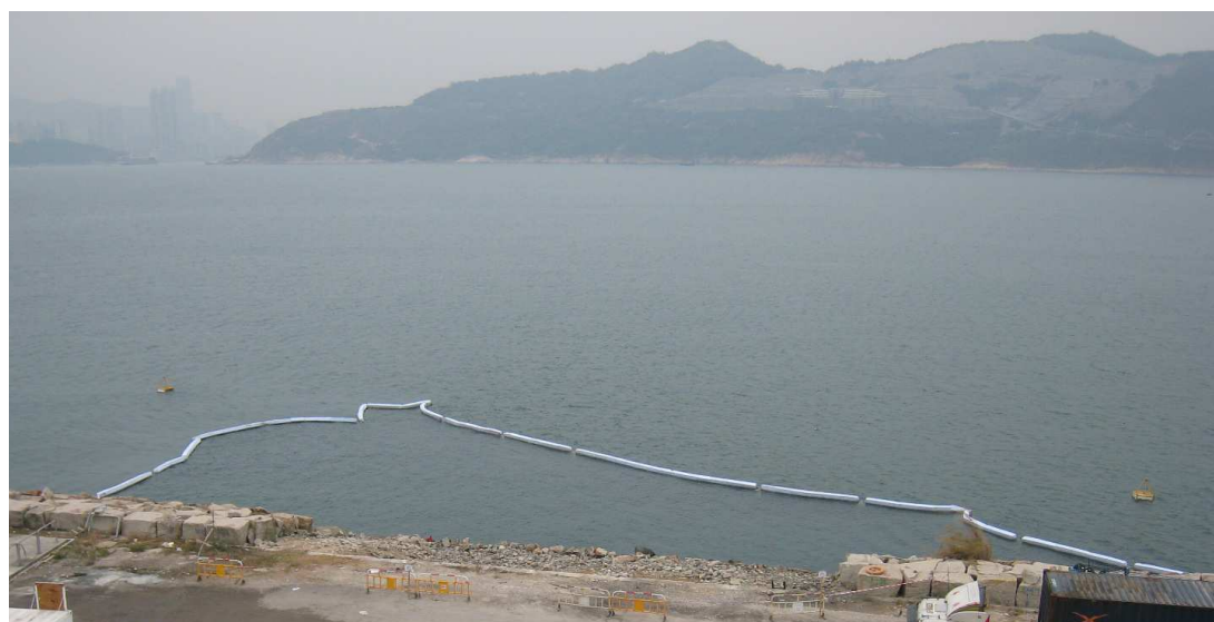
Figure 2 – Silt Curtain which Installed Onsite
