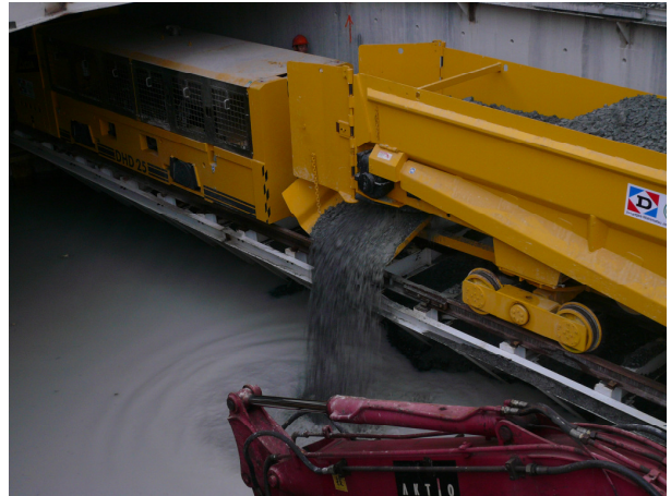
Photo 5: Shuttle car discharging excavated materials at the Adit Spoil Basin
