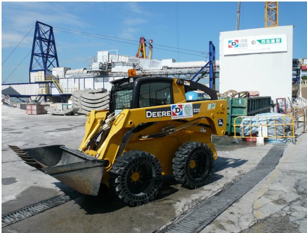
Photo 3: John Deere Skid Loader
