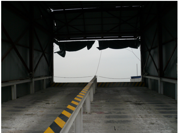
Photo 6: The Ramp Jetty
