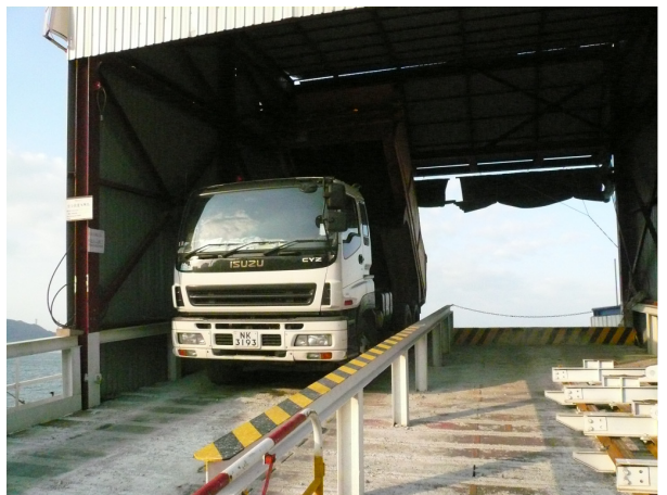
Photo 7: Dump truck discharging excavated materials onto the barge at the ramp jetty
