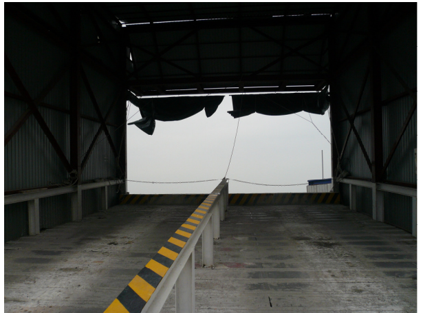
Photo 6: The Ramp Jetty
