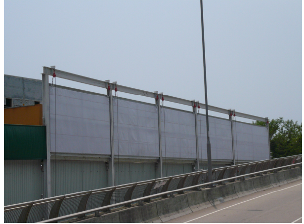
Photo 13: Noise barrier along Cyberport Road
