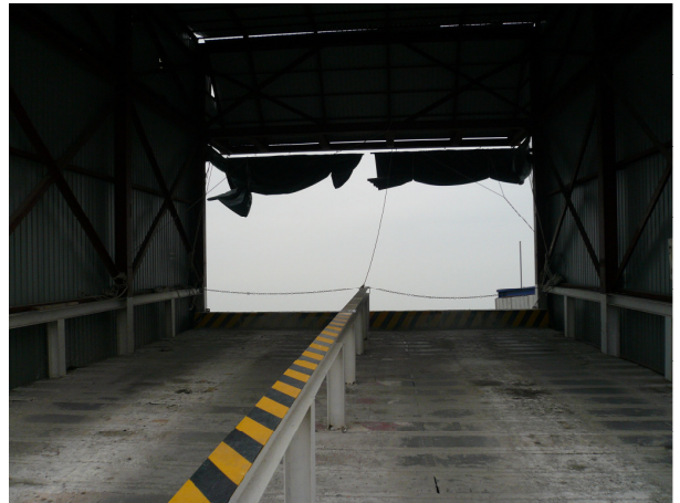
Photo 6: The Ramp Jetty
