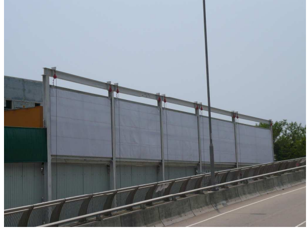
Photo 13: Noise barrier along Cyberport Road
