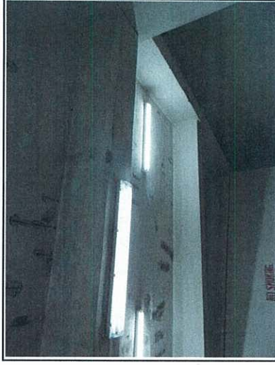
Photo 6: The ceiling of the Sub-Lower Ground Floor was concrete paved.
