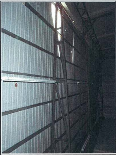
Photo 1: The ceiling of the Roof Floor was made of iron sheets.
