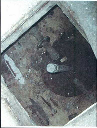
Photo 8: The top of the three kerosene tanks can be found after removal of three metal covers in the floor slab of Sub-Lower Ground Floor. No leakage found in the pipes connecting the tanks. No visual evidence of spillage/staining was observed.
