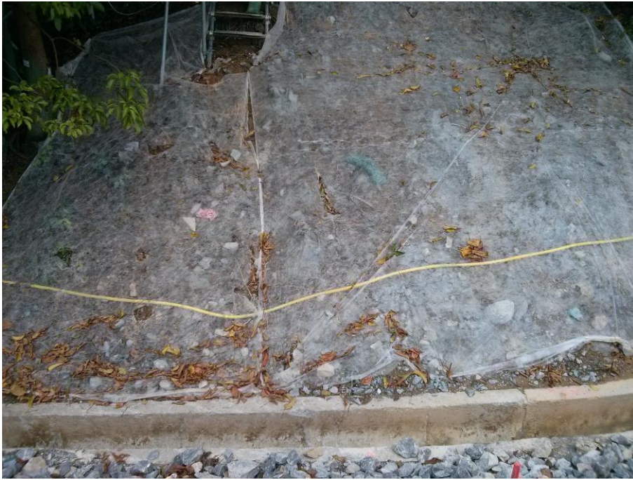
Hydro-seeding at unpaved slope nearby drainage
