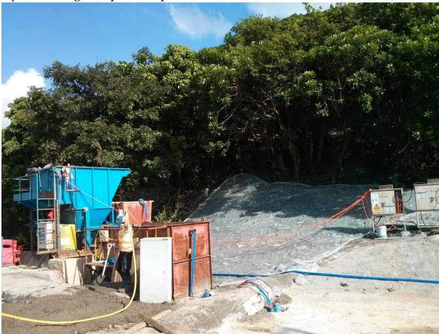
Hydro-seeding at unpaved slope
