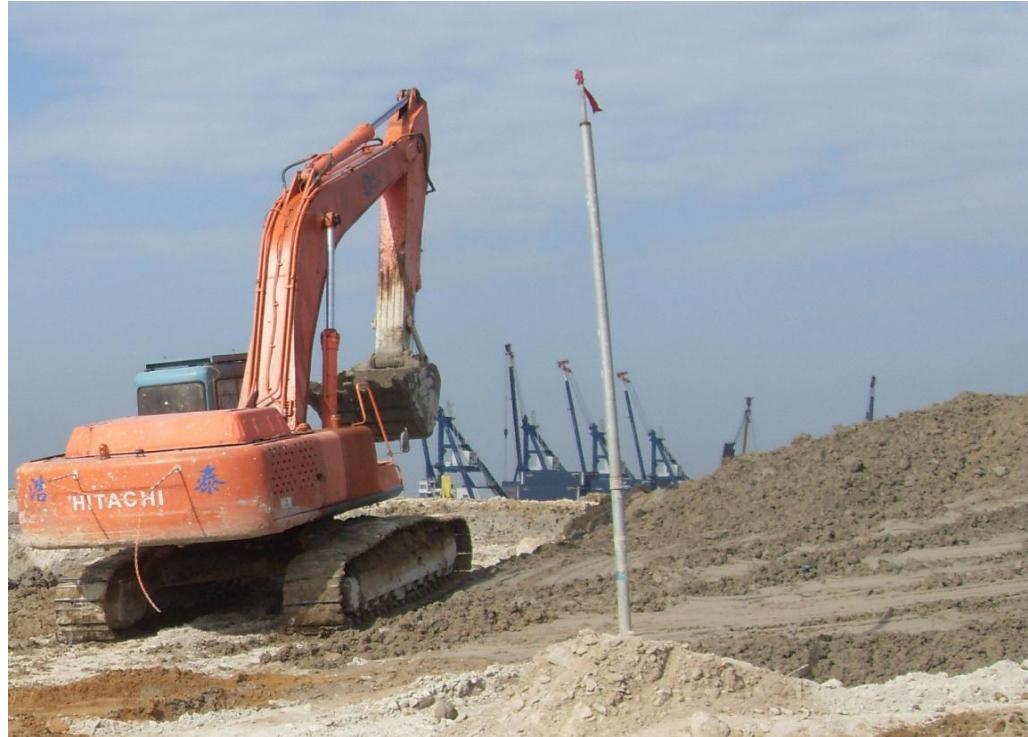
Stockpile was observed wet. (Reclamation Works Area - Portion N-C)
