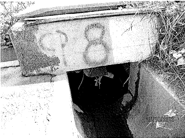
Photo 7 and 8 Catchpit No.8 Deposition of silt and silty water are found at Catchpit No.8 at CREO. The Contractor is reminded to frequently clean and maintain the catchpit.
