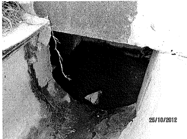
Photo 7 and 8 Catchpit No.8 Deposition of silt and silty water are found at Catchpit No.8 at CREO. The Contractor is reminded to frequently clean and maintain the catchpit.
