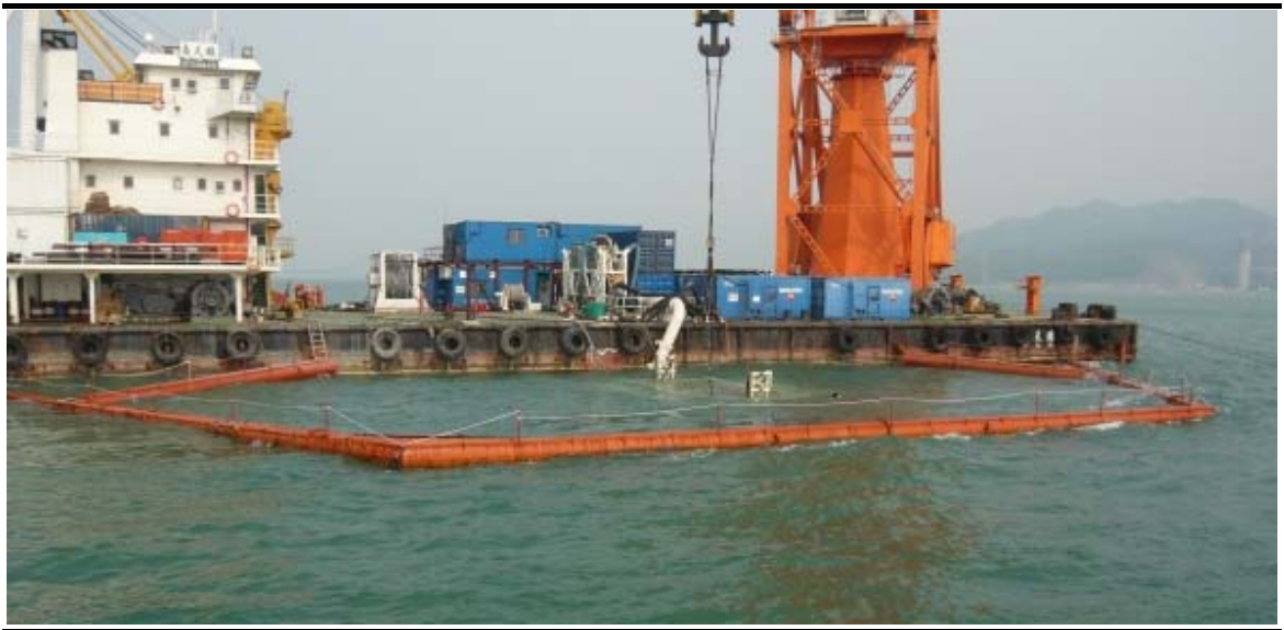
Figure 2. Silt Curtain for Jetting Machine
