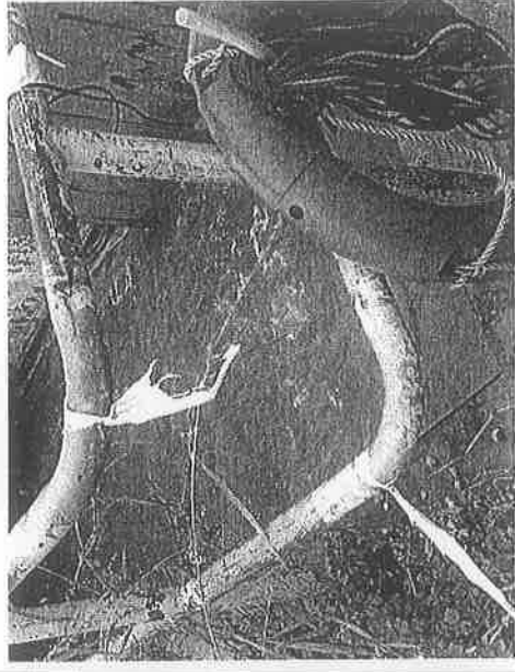
Photo 161017_005 (Discharge point close to sea wall)
