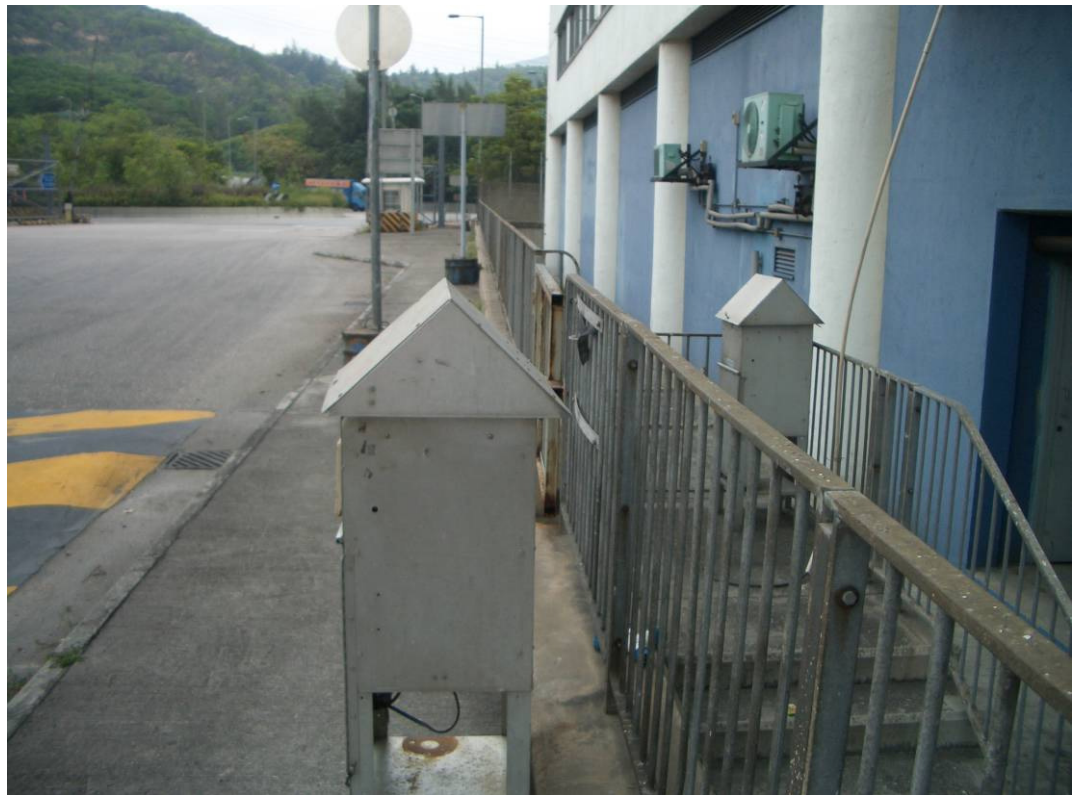
AM2 - River Trade Terminal Office
