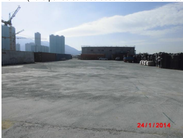
View B (Hard paved surface observed at Works Area WA2)
