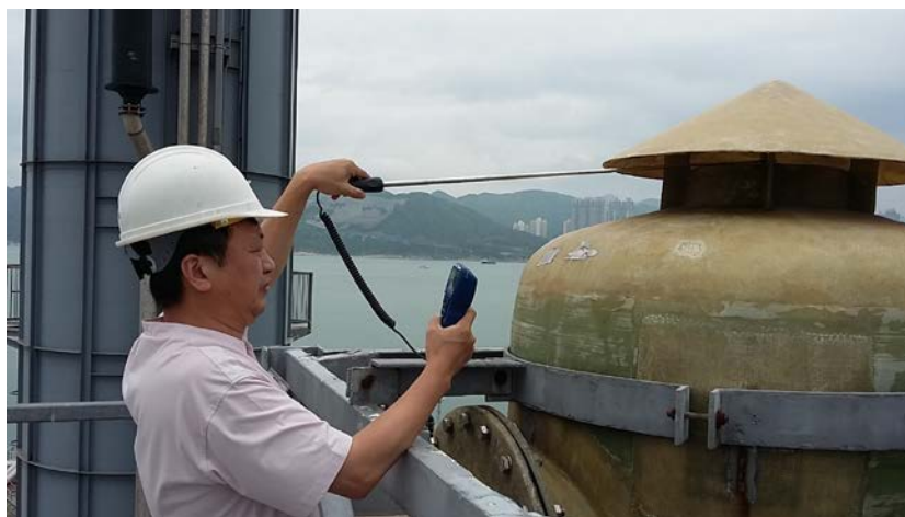
Final air scrubber
