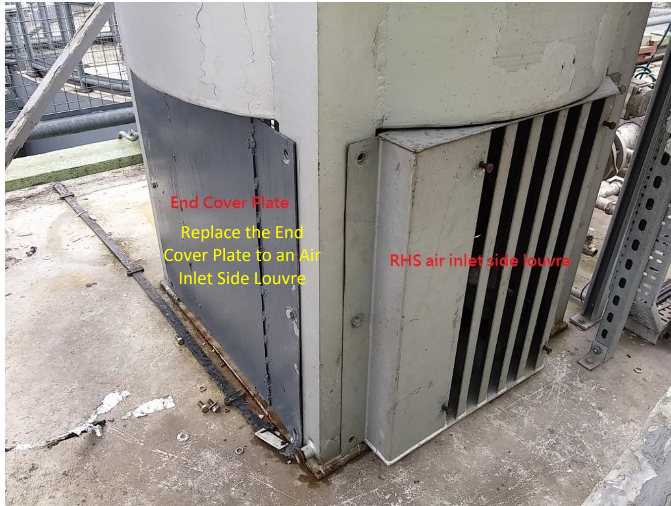
Figure 2: Recommended Changes (in yellow) on the Air-Intake Point of the Biogas Flare Stack
