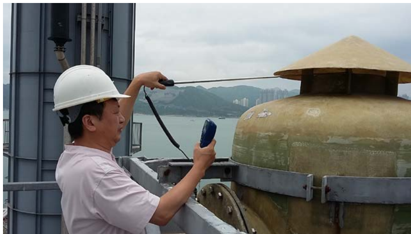
Final air scrubber
