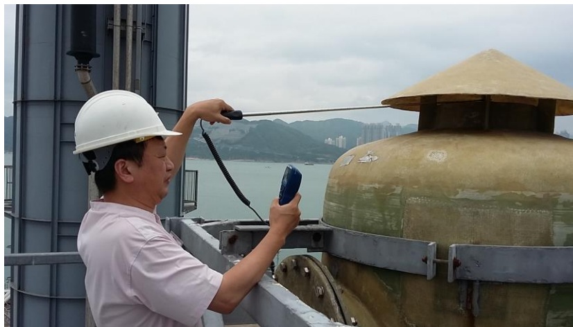
Final air scrubber
