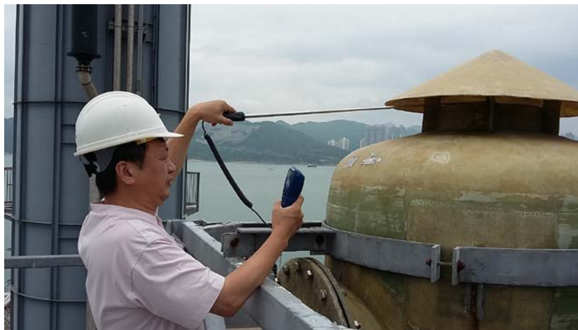
Final air scrubber
