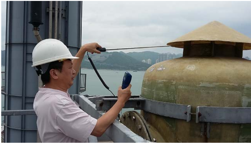
Final air scrubber
