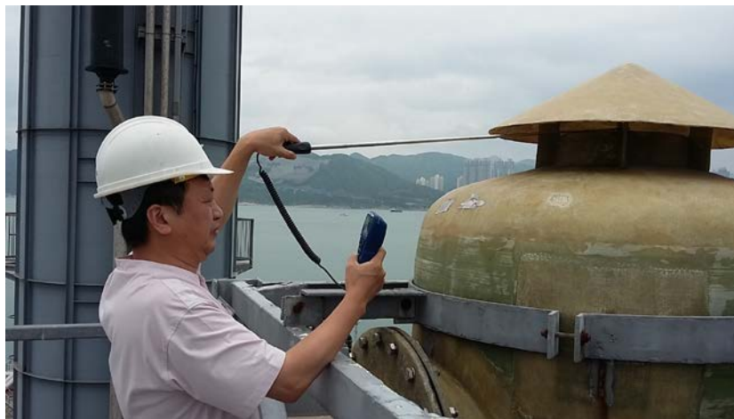
Final air scrubber
