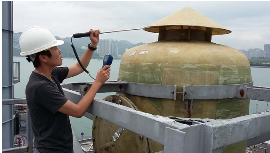
Final air scrubber
