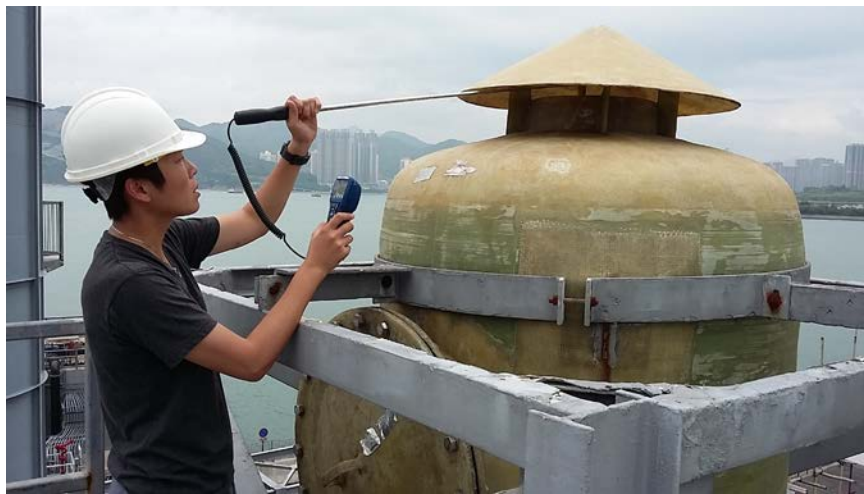
Final air scrubber
