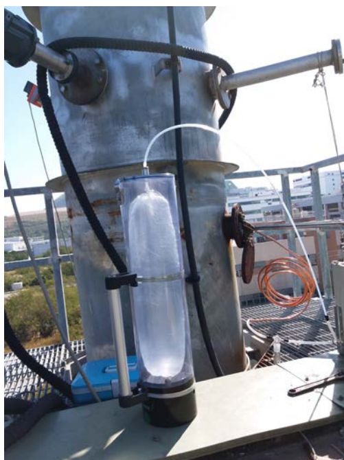
Boiler stack (EP2)
