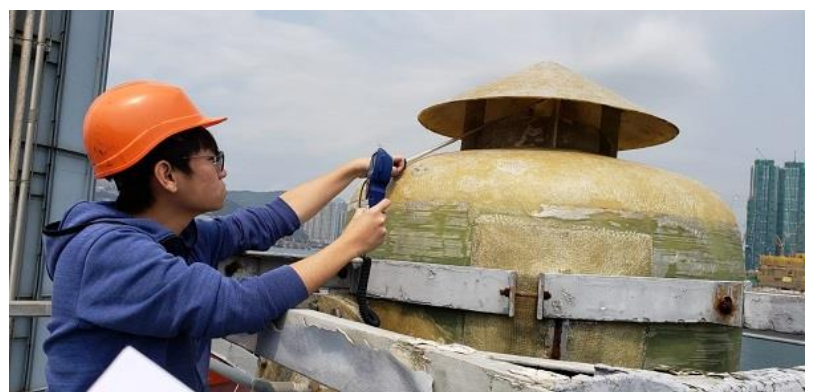
Final air scrubber
