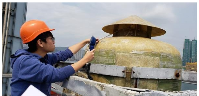
Final air scrubber
