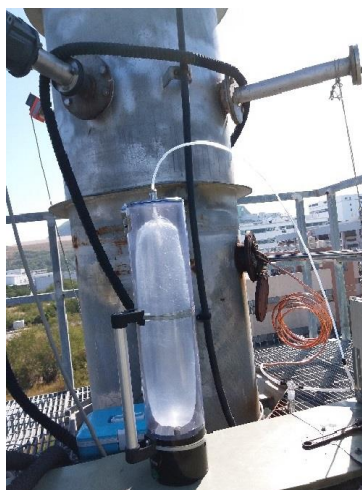
Boiler stack (EP2)
