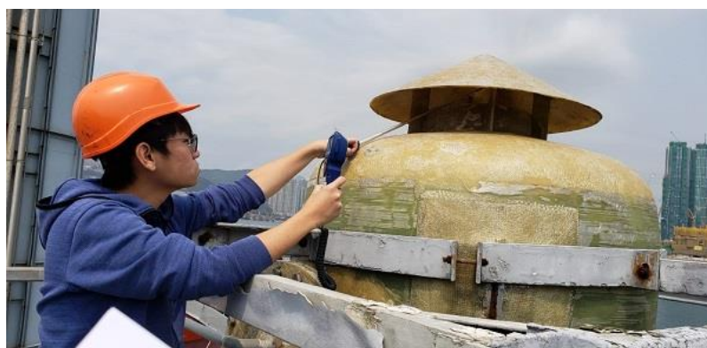
Final air scrubber
