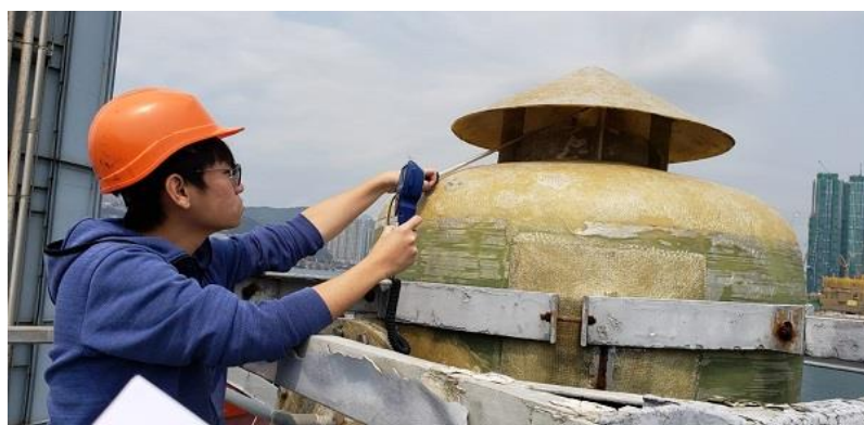
Final air scrubber
