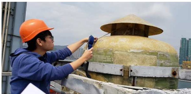
Final air scrubber
