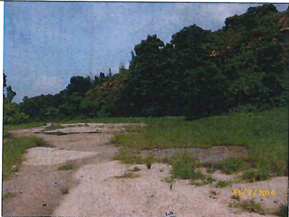
General view of works area D
