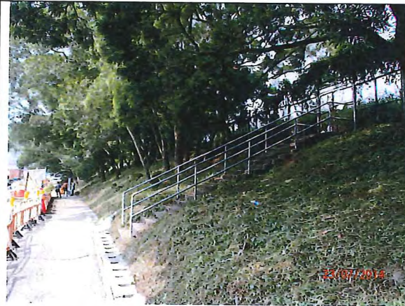
General view of works area B at northern bound of Lung Mun Road (opposite to Butterfly Beach Laundry)
