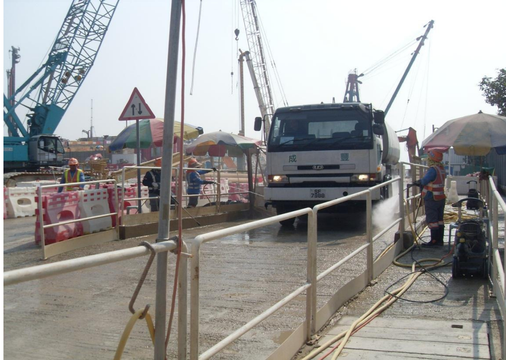
Wheel washing facilities is adequately maintained. (Site entrance at Reclamation Works Area)
