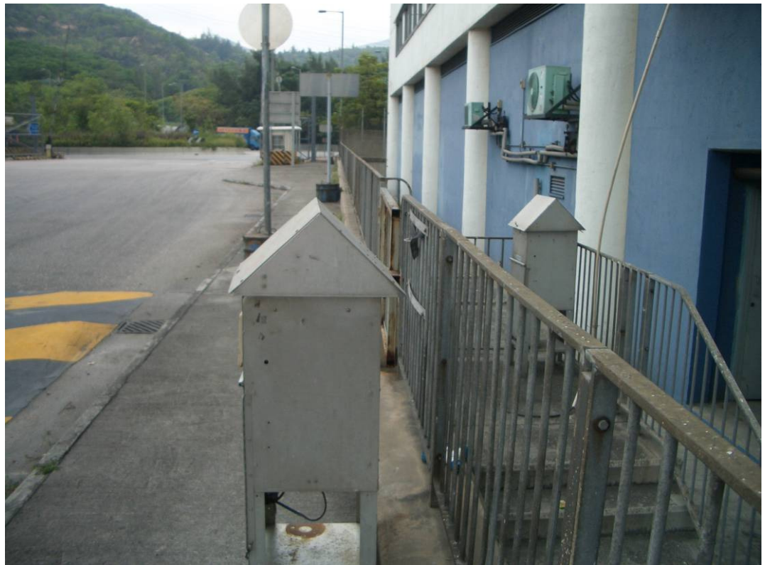
AM2 - River Trade Terminal Office
