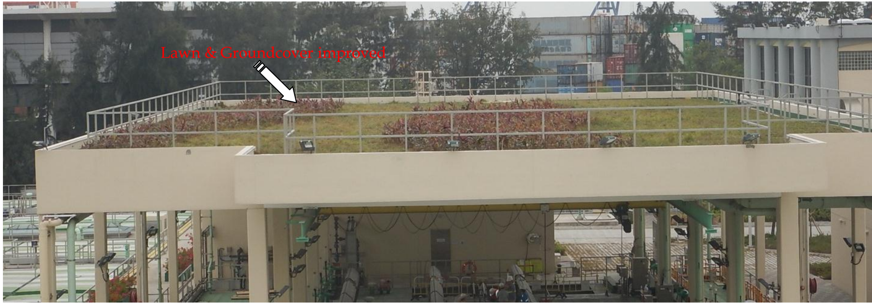
Photo no. F-01 : Lawn and groundcover at roof floor were observed improved.
