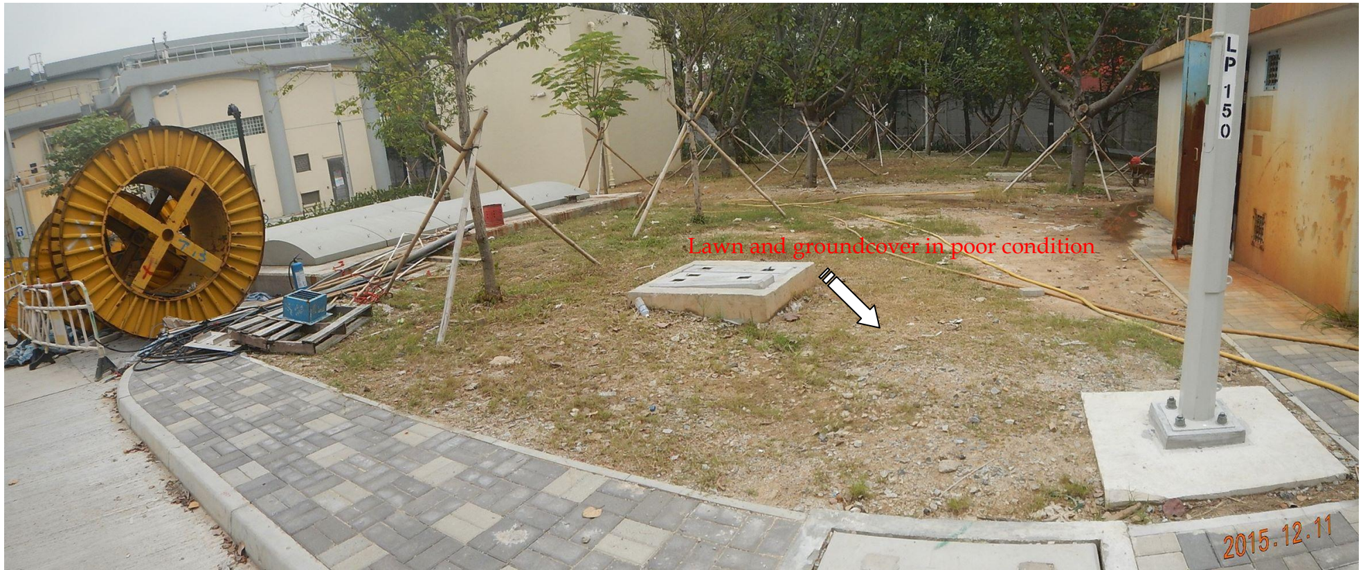
Photo no. G-05: Lawn and groundcover were observed in poor condition.
