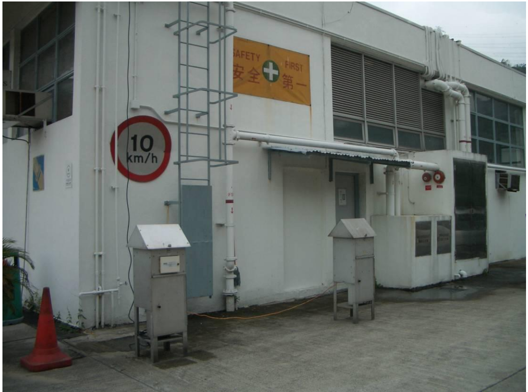
AM1 - Tuen Mun EMSD Servicing Vehicle Station
