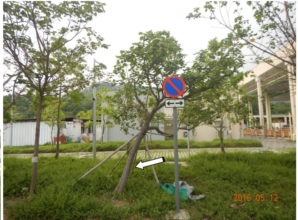
Leaning tree observed
