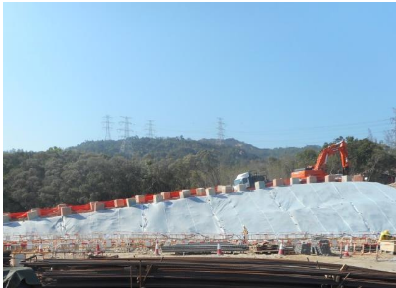
Item 4. Sheeting of soil stockpile was provided.
