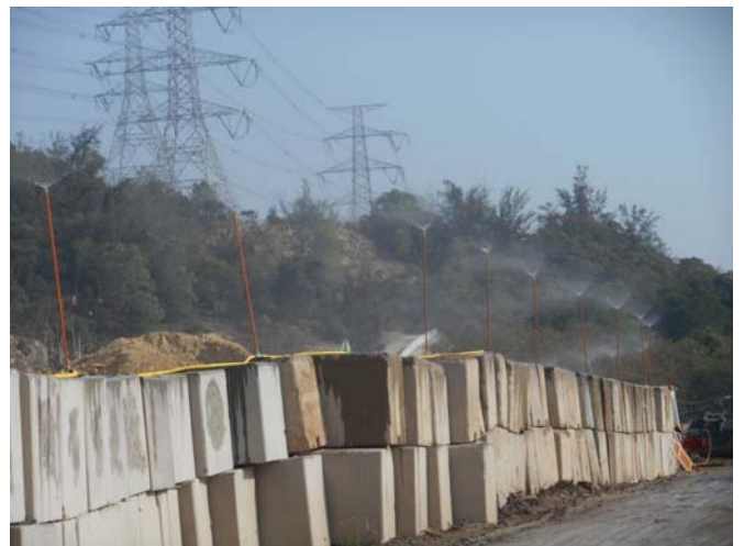
Photo 2 Installation of auto-water sprinkler in dusty area
