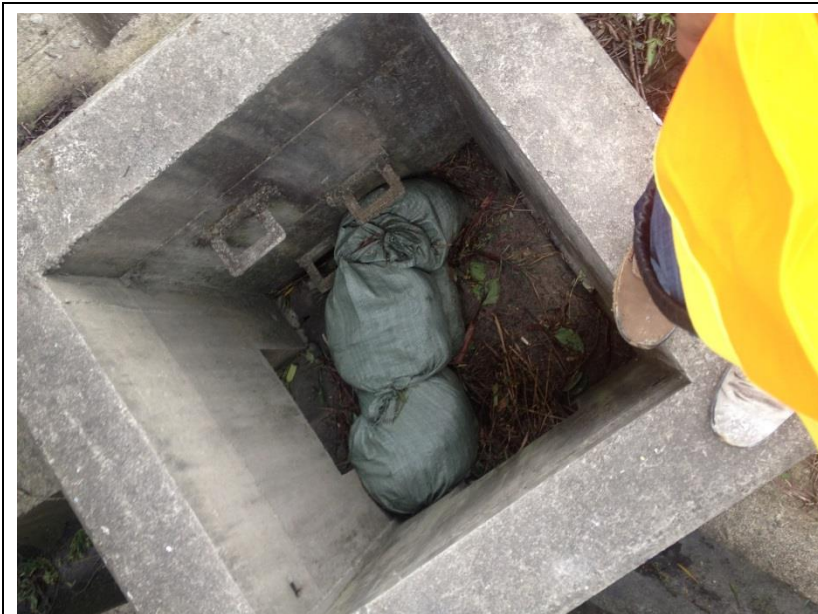
Item 7. Ensure no run-off into water body.
