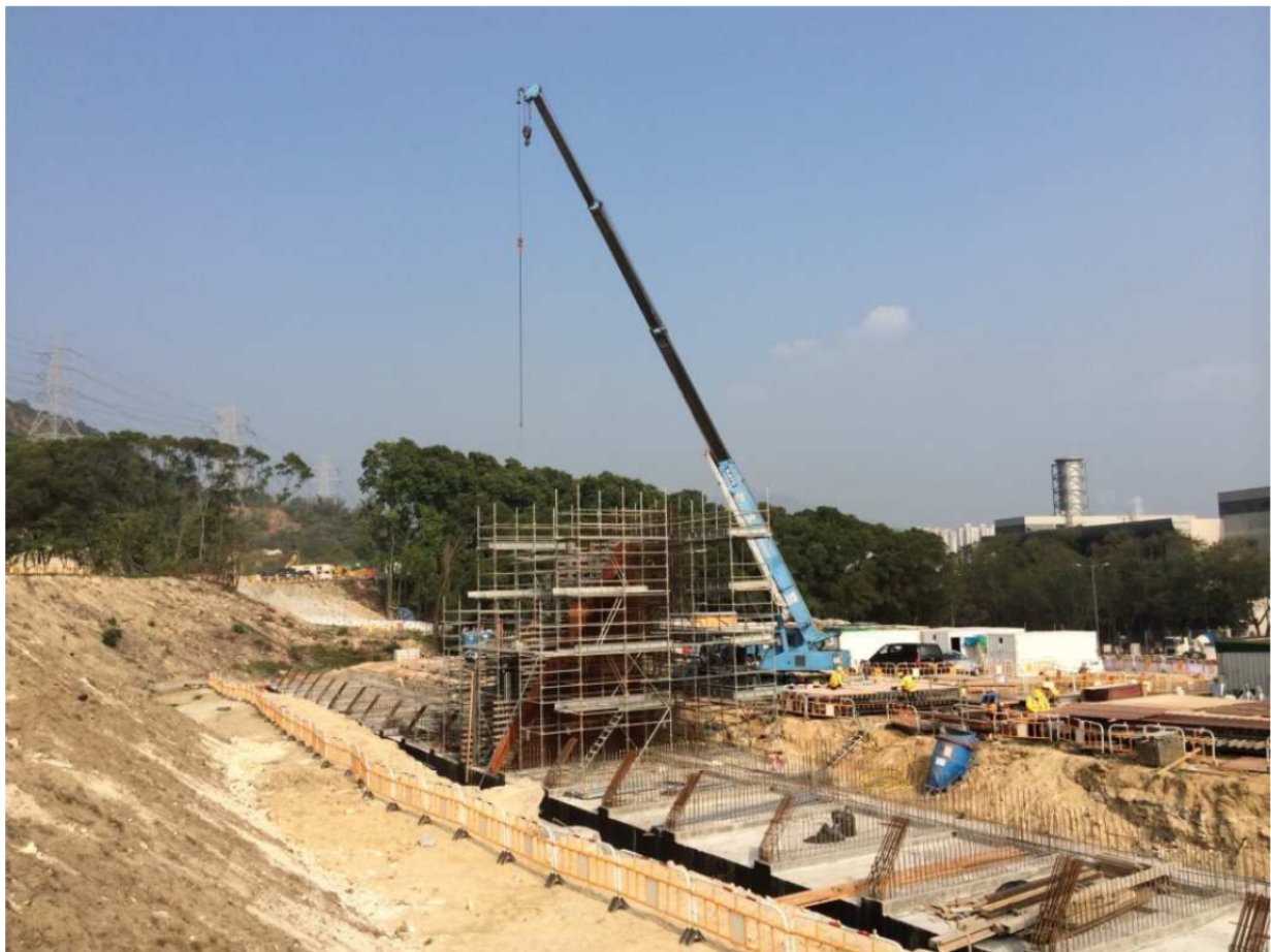
Landfill Gas Monitoring Location – Retaining Wall F
