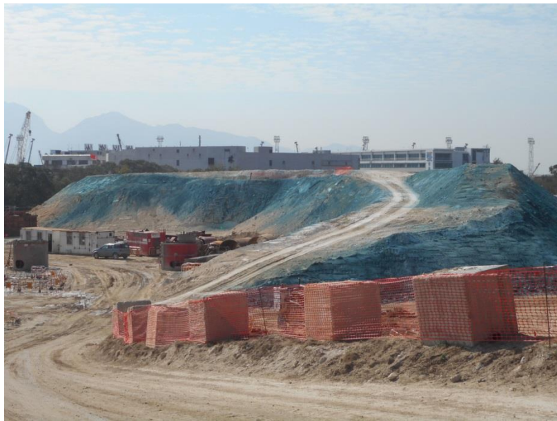
Item 4. Hydro-seeding of soil stockpile was provided.
