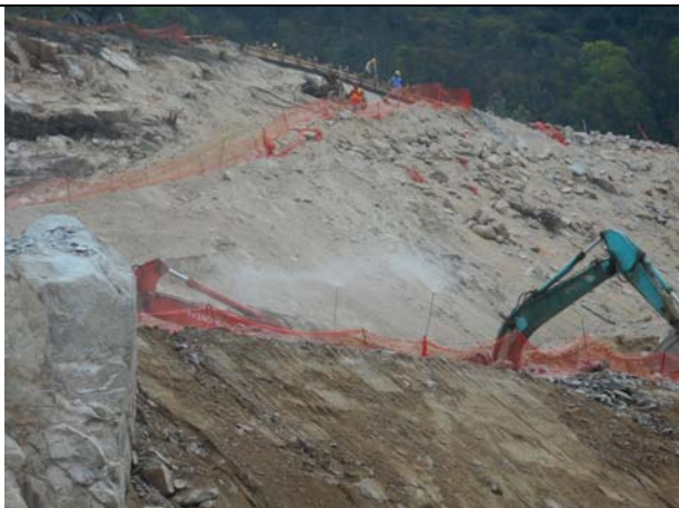
Photo 5 Installation of auto-water sprinkler in dusty area
