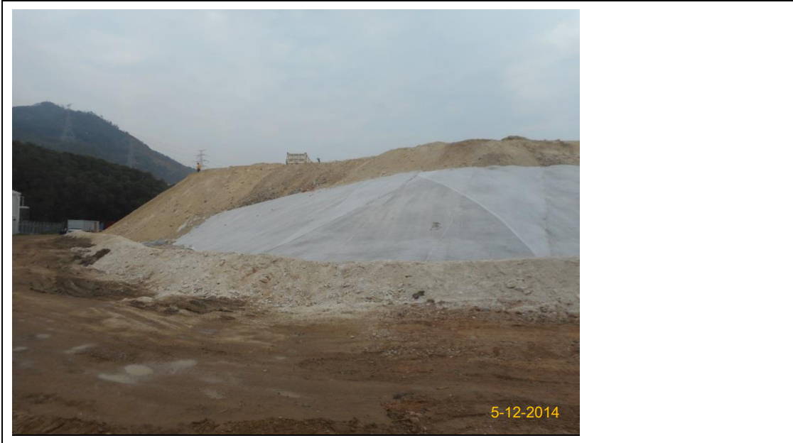
Item 4. Hydro-seeding provided at stockpile.
