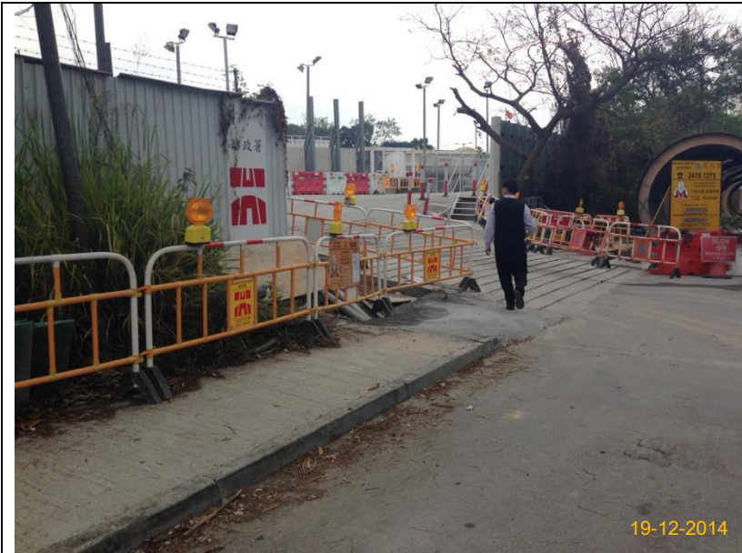
Item 5. Hoardings around works area.
