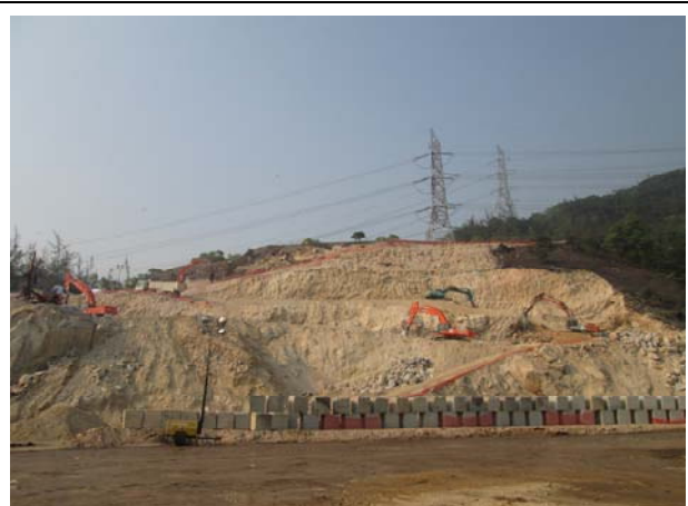
Photo 8 Wetted haul road was observed on 12 December 2014.
