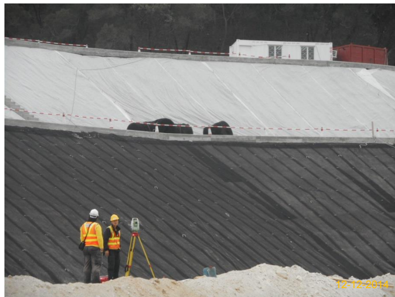
Item 4. Hydro-seeding or sheeting provided at stockpile.
