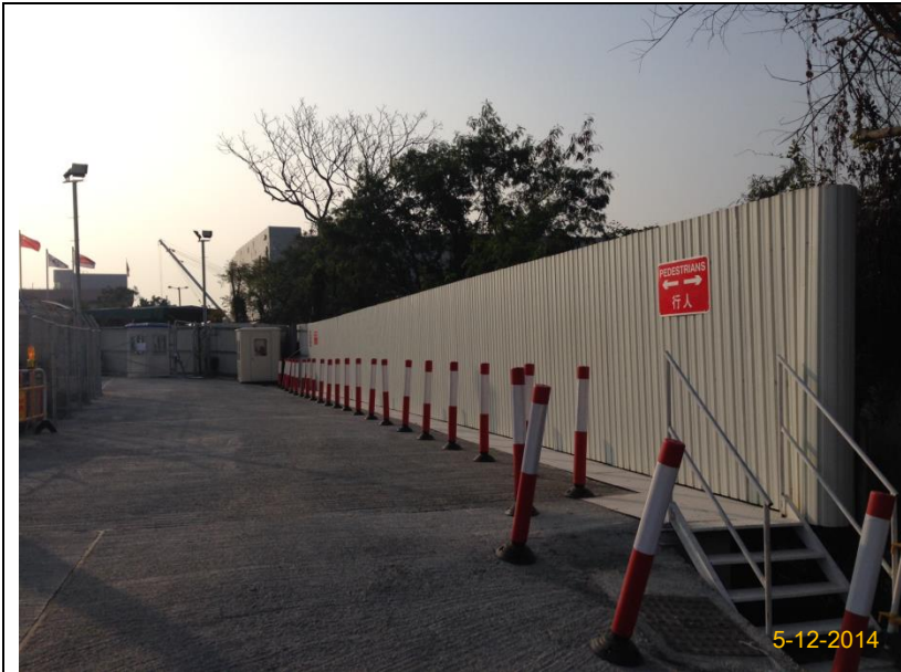
Item 5. Hoarding around works area.
