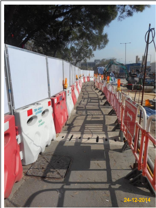
Item 5. Water Barrier with panel around works area.
