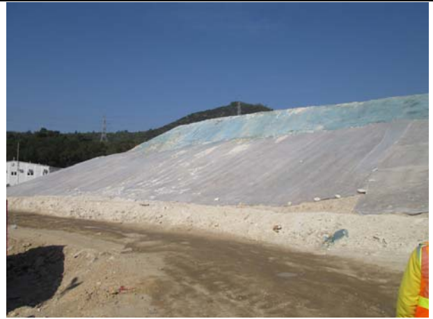
Photo 7 Covering of the exposed slopes by geotextile net was observed on 17 December 2014.
