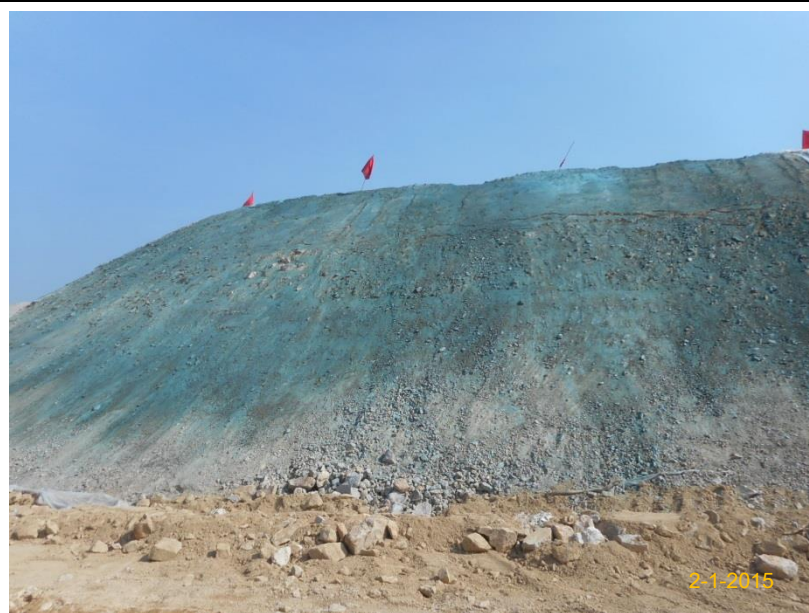
Item 4. Hydro-seeding provided at stockpile.
