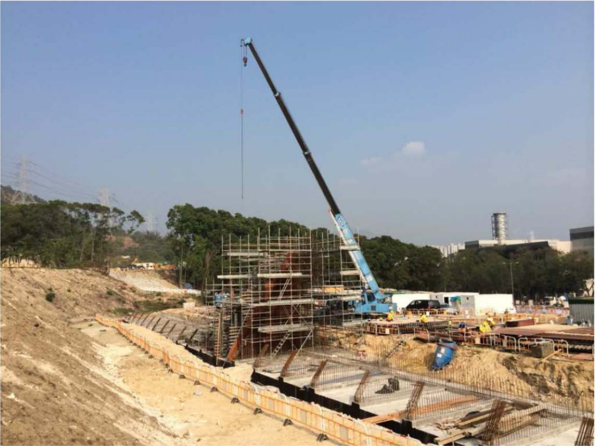
Location of the Retaining Wall F
