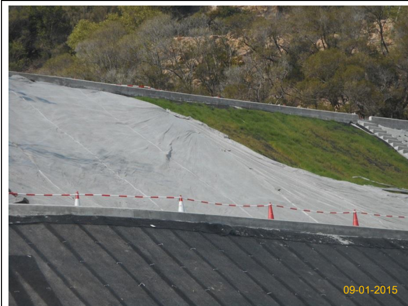
Item 4. Hydro-seeding or sheeting provided at stockpile.
