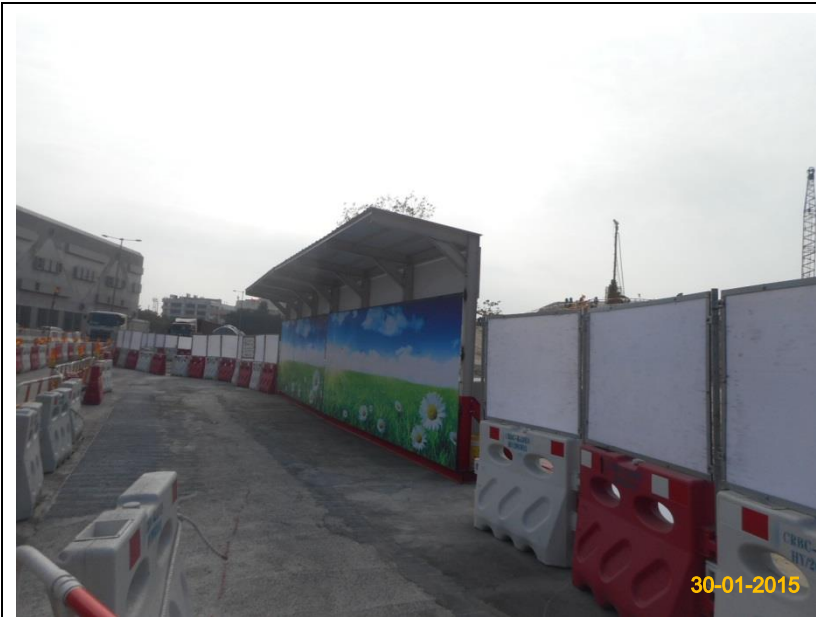
Item 5. Water Barrier with panel around works area.
