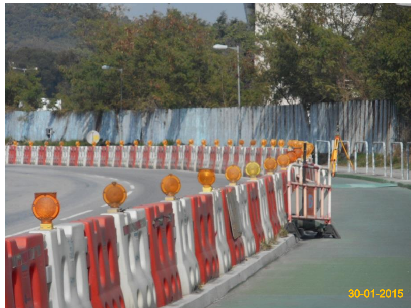
Item 6. Temporary traffic management lighting.
