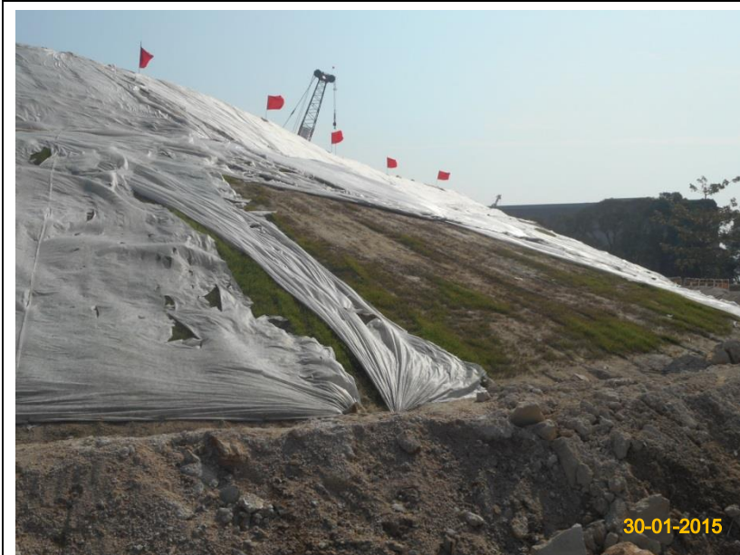
Item 4. Hydro-seeding or sheeting provided at stockpile.
