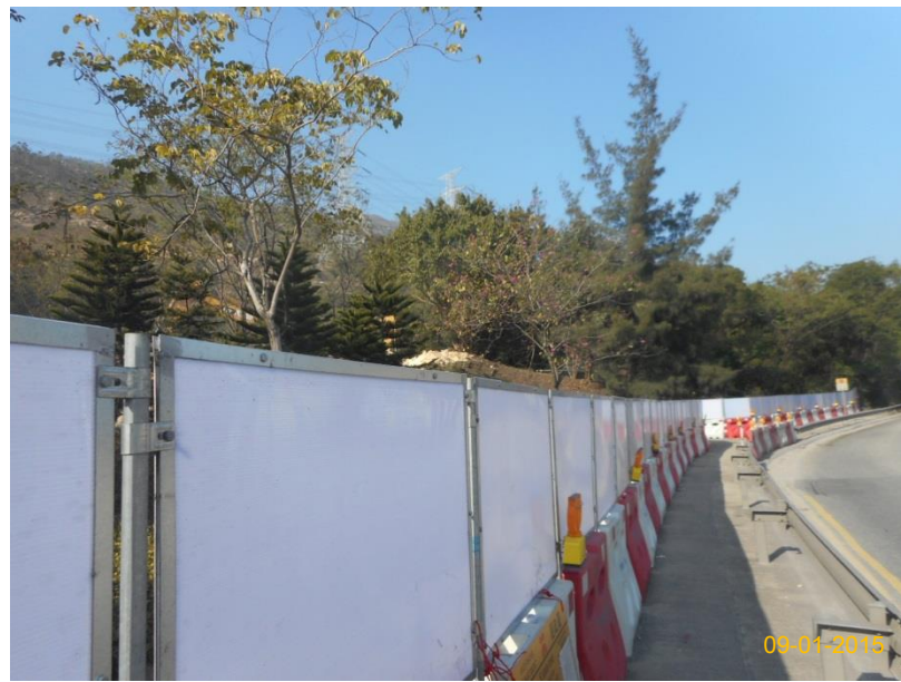
Item 5. Hoarding around works area. Item 6. Temporary traffic management lighting.
