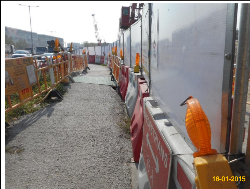
Item 5. Hoardings around works area. Item 6. Temporary traffic management lighting.
