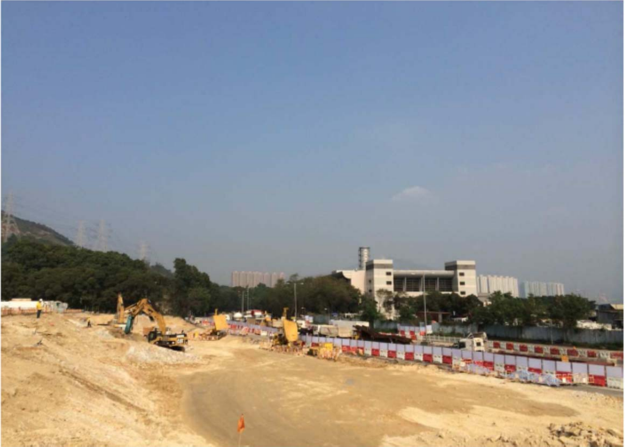
Location of the Retaining Wall B
