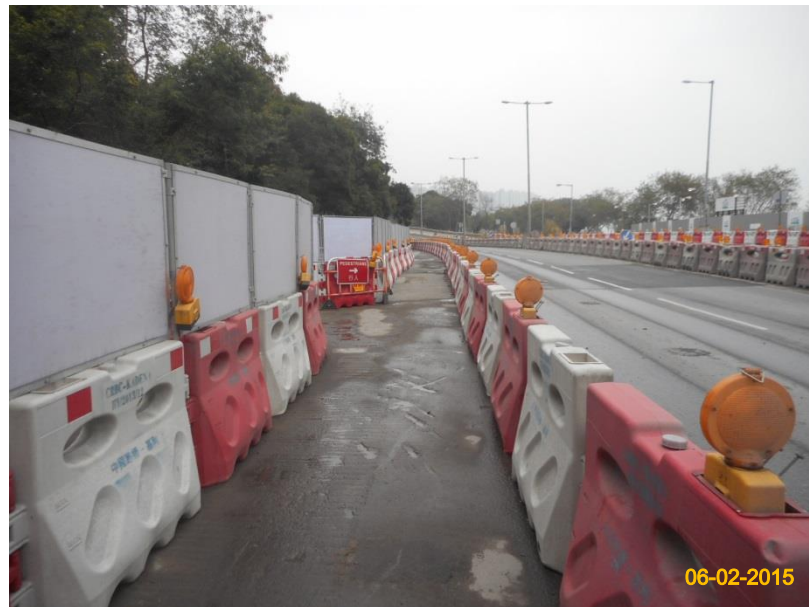
Item 6. Temporary traffic management lighting.
