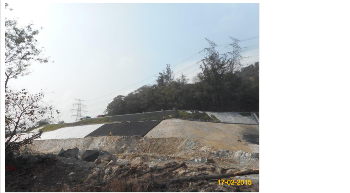
Item 4. Hydro-seeding or sheeting provided at stockpile.
