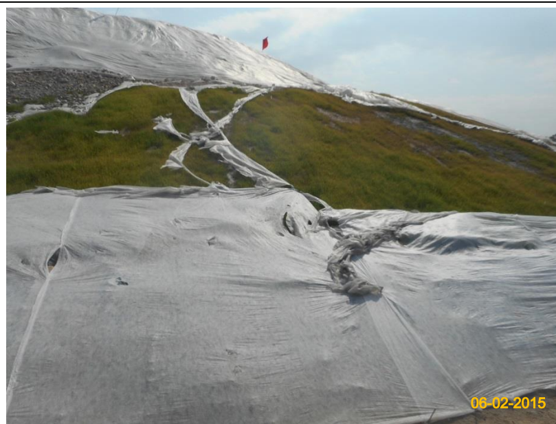
Item 4. Hydro-seeding or sheeting provided at stockpile.
