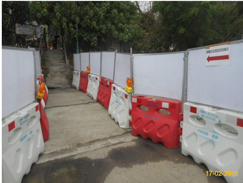
Item 6. Temporary traffic management lighting.
