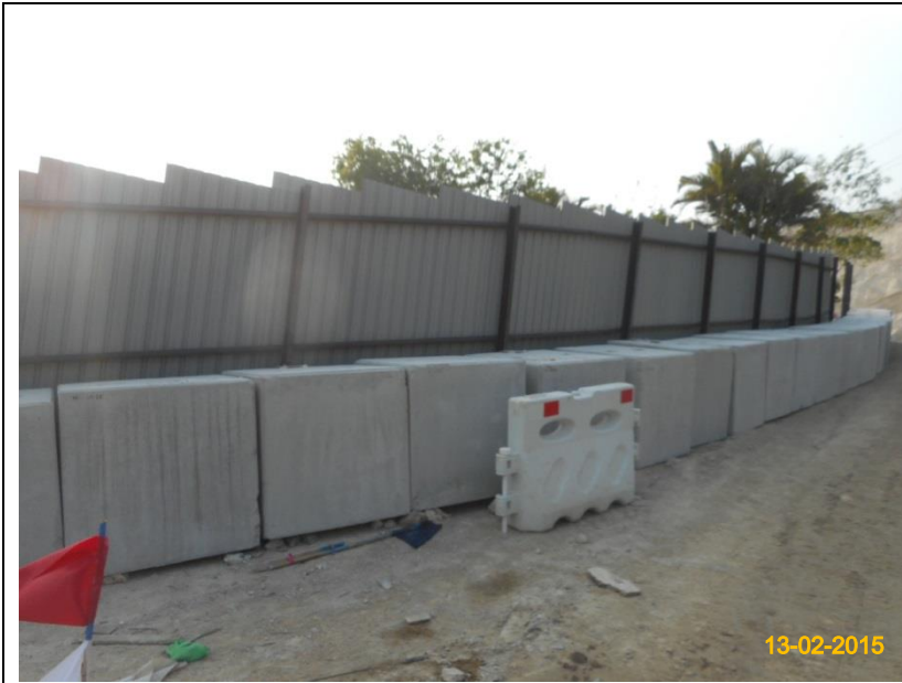
Item 5. Hoarding with panel around works area.
