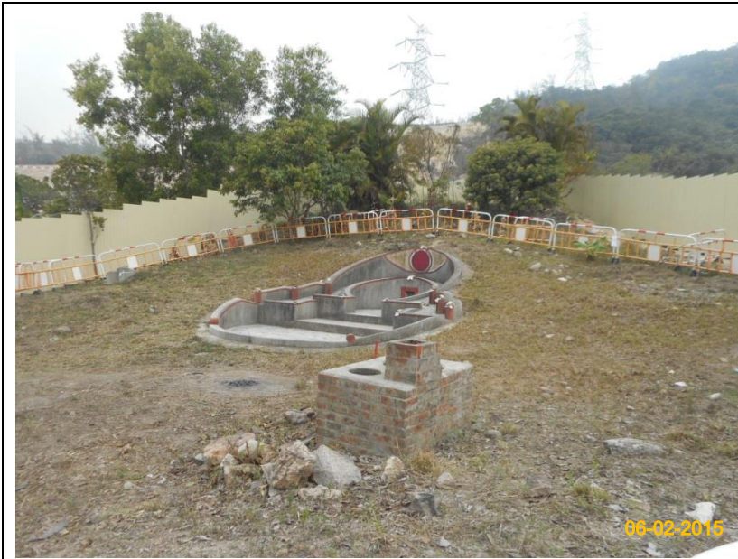
Item 5. Hoarding with panel around works area.
