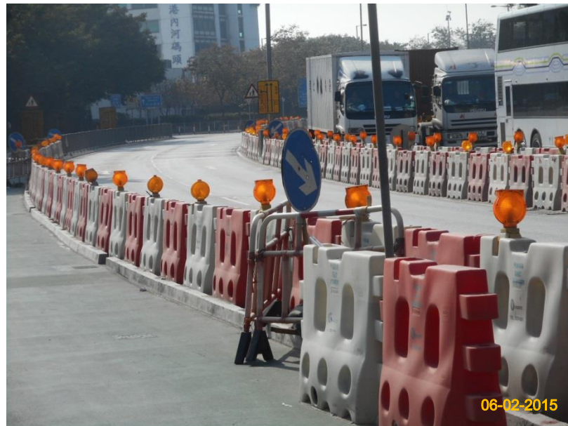
Item 6. Temporary traffic management lighting.
