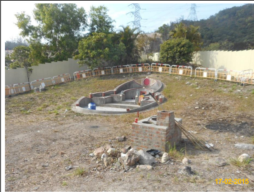
Item 5. Hoarding with panel around works area.
